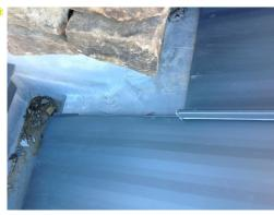
General - Failing Penetration (Remedial) Quantity: 2147483647 EA Deficiency: Improper flashing. Corrective Action: The penetration should be repaired/flashed per industry standards to ensure a water tight seal.
