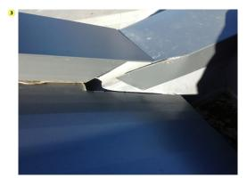
Metal Roof - Ridge/Hip - Zee Closure - Caulk Vertical Leg (Remedial) Quantity: 2147483647 EA Deficiency: Needs to be closed off with zee closure and flashing. Corrective Action: Caulk all vertical legs of Zee Closure.
