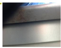
Metal Roof - Panel - Panels-Seam Fully (Remedial) Quantity: 2147483647 EA **Deficiency:** Panels need to be fully engaged onto drip edge. Check all **Corrective Action:** Fully seam panels to insure watertightness. Using hands camer.
