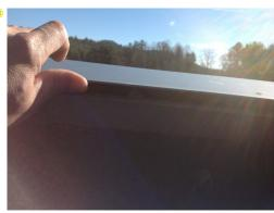
Metal Roof - Ridge/Hip - Rivets-Needed (Remedial) Quantity: 2147483647 EA **Deficiency:** Rivets need to be added where ridge is not locked onto zee closure. **Corrective Action:** Add rivets at the ridge and hip.
