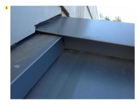
Metal Roof - Ridge/Hip - Zee Closure - Caulk Vertical Leg (Remedial) Quantity: 2147483647 EA Deficiency: Vertical Legs of Zee Closure is not caulked. Check all. Corrective Action: Caulk all vertical legs of Zee Closure.
